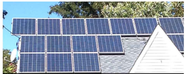
Panels are over the edge
