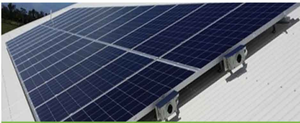
Panels are installed within the edge of the roof
